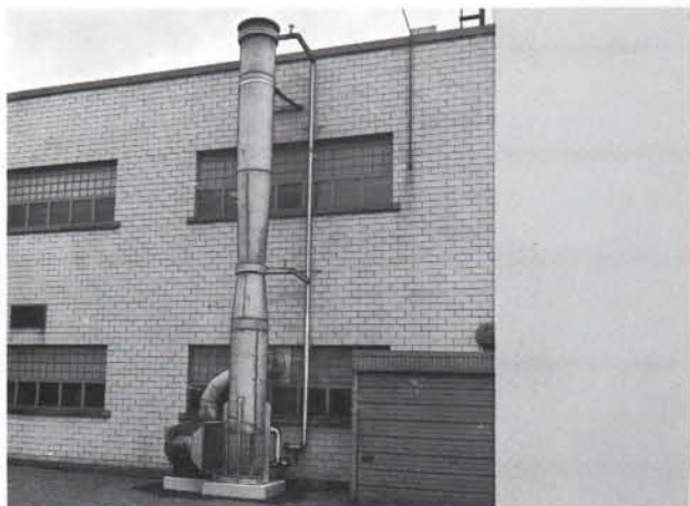
Water-wash design Induction Venturi being used to exhaust perchloric acid fumes from major Canadian Steel plant.
